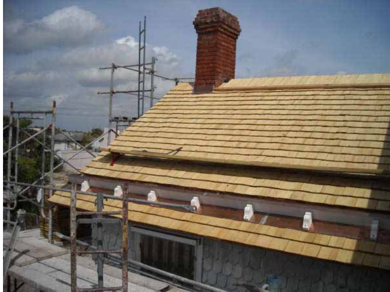
Shingled Roof & Stop Gutters South Side Shown
