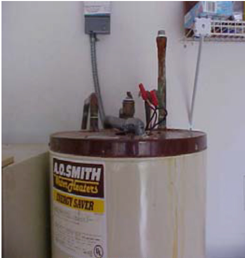
Figure 6 - Before. Old, rusted, electric water heater.
