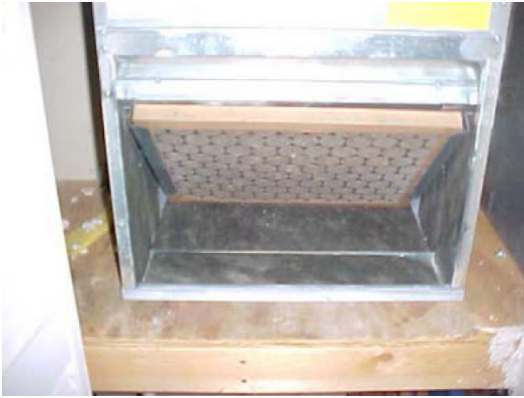
Figure 1 - Air conditioner filter inside open unit.
