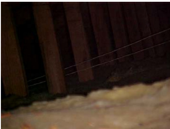
Figure 2 - Before. Attic insulation is matted and old.
