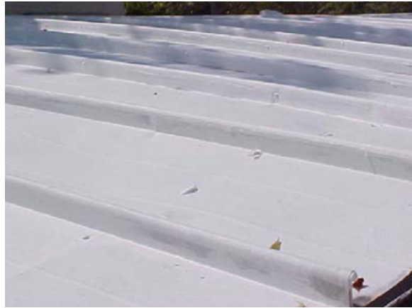
Figure 13 - After. Roof treated with coating.
