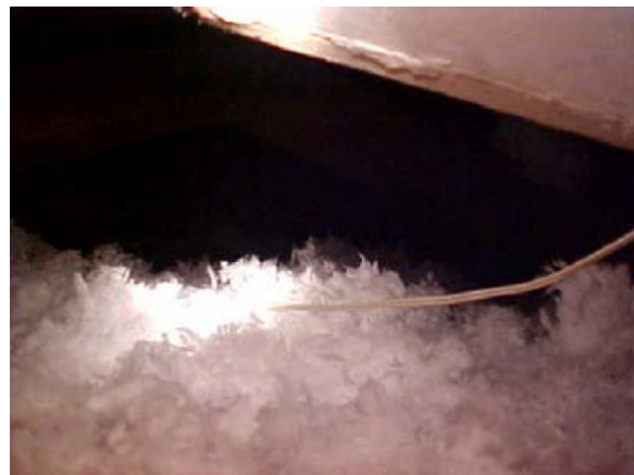
Figure 3 - After. Attic insulation is loose and fluffy.
